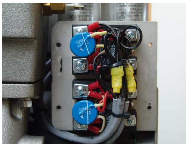
Fig. A.3.6-22: Solid state relays for booster capacitors 120V/60Hz
